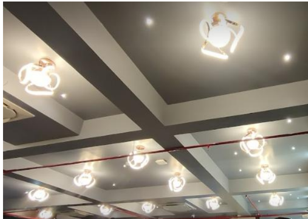
Figure 3. Artificial lightings along the ceiling slab at 'Masala Marke' Source: (Parikh K, 2024)
