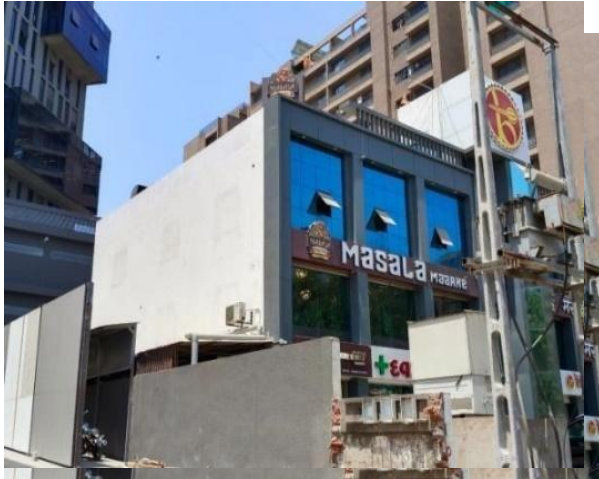
Figure 1. Blank concrete wall at 'Masala Marke' facing southwest Source: (Parikh, 2024)
